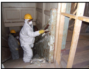
Workers removing lead paint.
